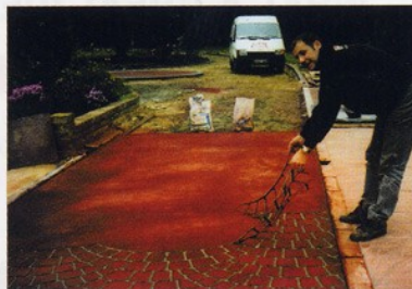
Step 8 Remove Stencil pulling evenly - revealing the pattern, with contrasting colour joints.
