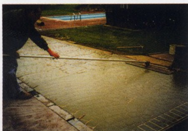
Step 4 Apply stencil over remaining area and float into surface.
