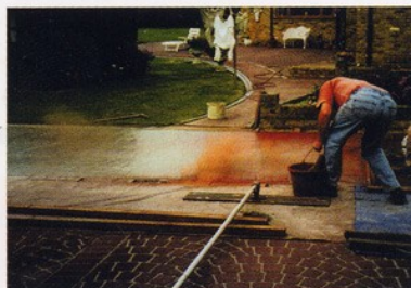
Step 5 Apply PERMACOLOUR colour hardener.
