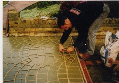
Step 3 Apply chosen pattern Stencil - aligning and trimming to size.
