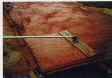
Step 6 Float PERMACOLOUR into the surface.
