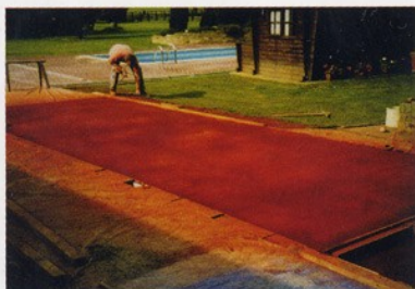
Step 7 Final coat can be left un-floated to give decorative anti-slip finish (if required).
