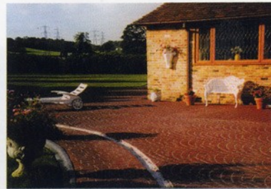
Step 9 Finished area.
