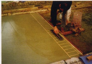
Step 2 Float Stencil Border into the surface using a trowel.
